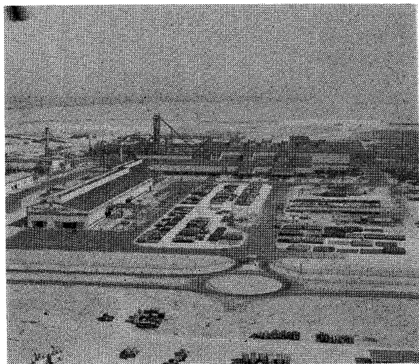
写真1 Overall view of QASCO.
