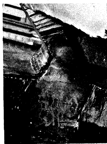
Photo. 4 Lamellar tearing occurred at the opposite side plate and propagated to the toe
